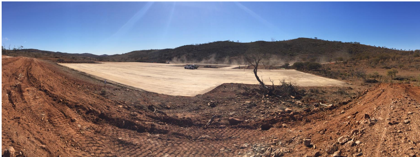
Silverton Wind Farm Substation Bench Completed
