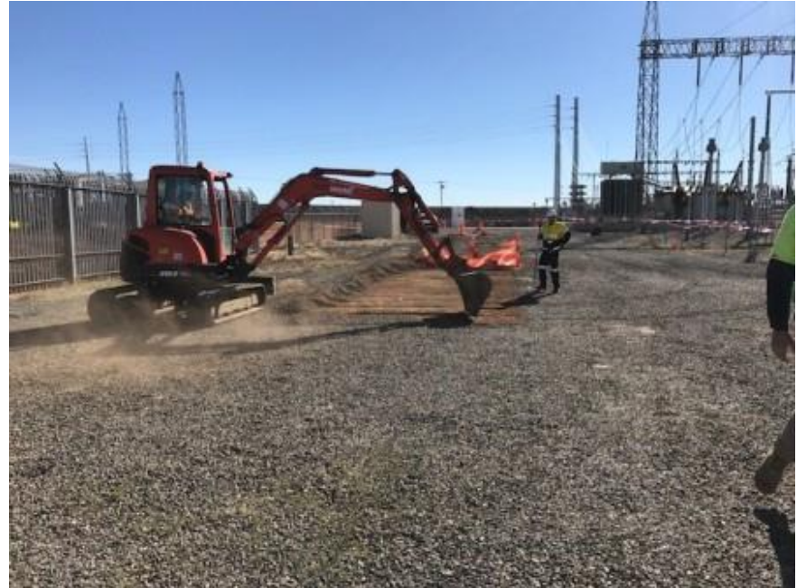
Works at existing Broken Hill 220kV Substation
