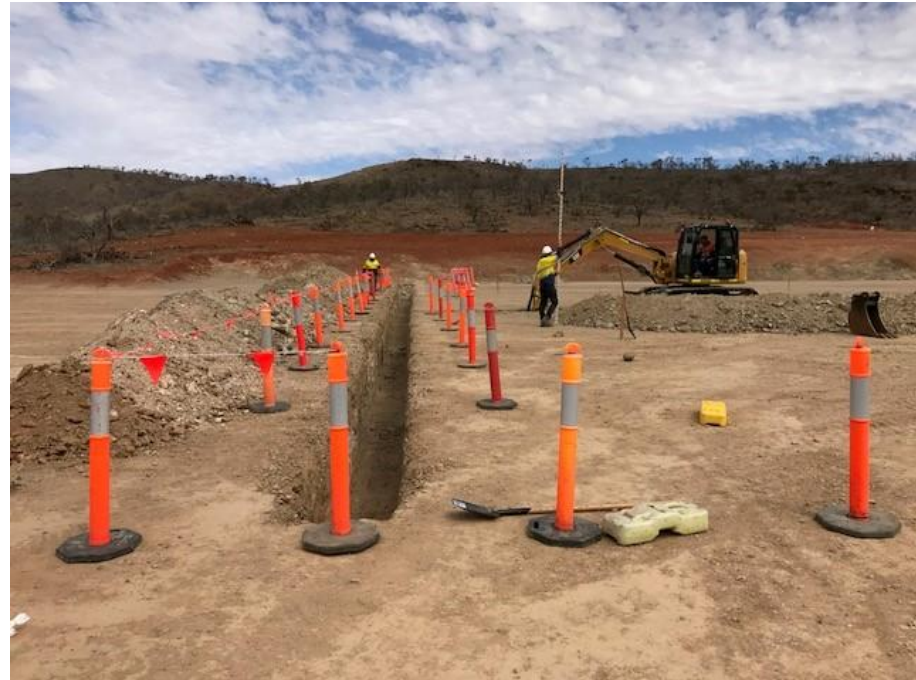
Works at new Silverton Substation
