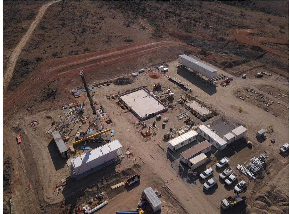
Works at new Silverton Substation
