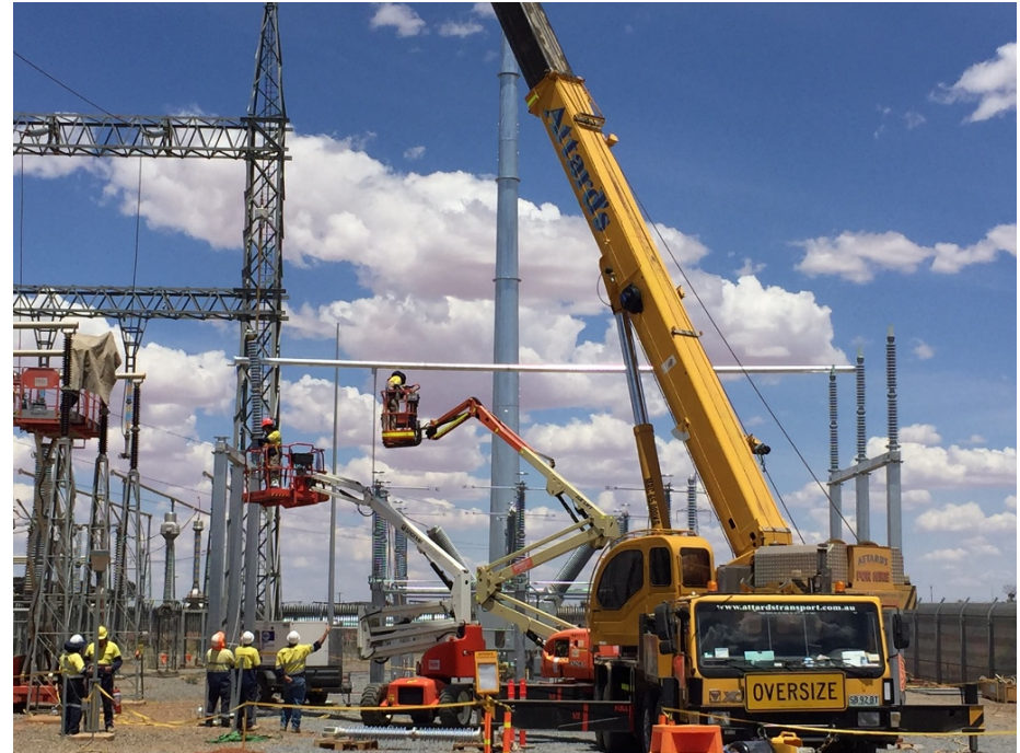
Works at existing Broken Hill 220kV Substation
