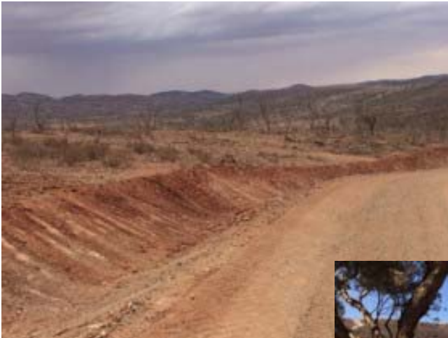
(Above) Installed spoon drains (Right) Installed cross drain (Far Right) Installed spoon drains
