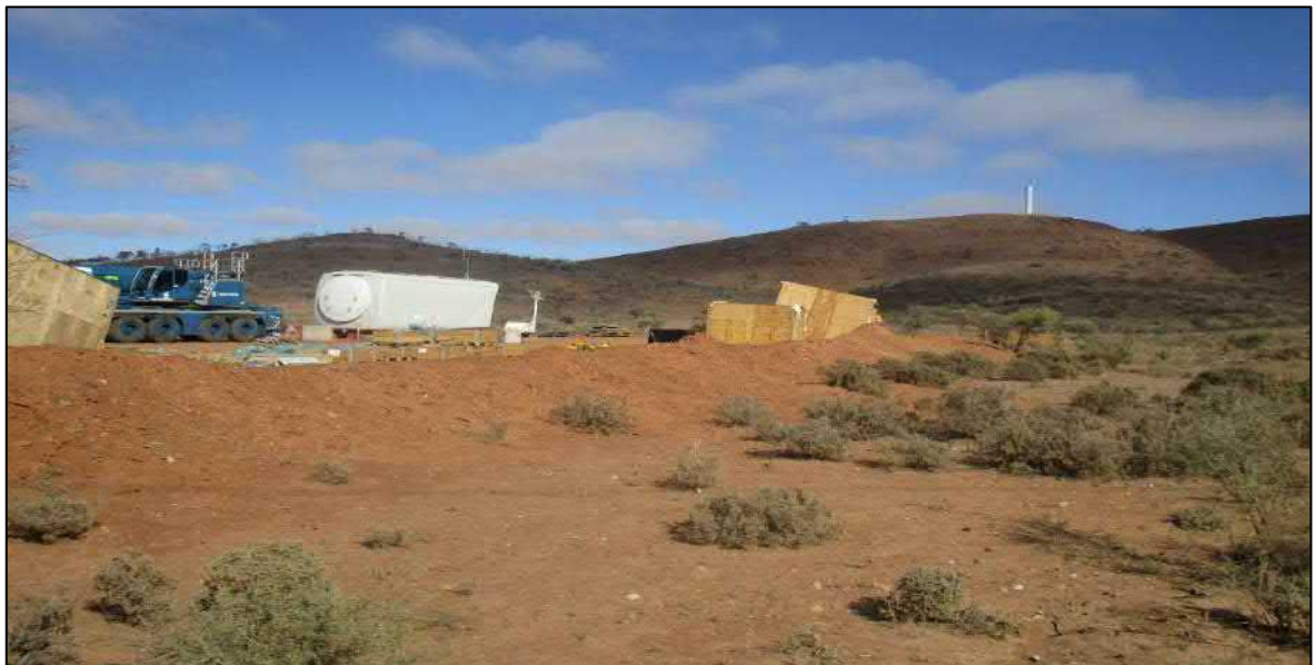
Photo: Equipment laydown area with stockpiled topsoil, awaiting rehabilitation.
