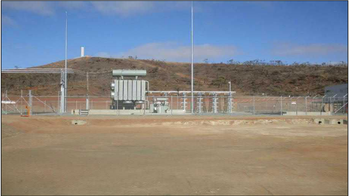
Photo: Electrical Substation, with rehabilitation works commenced.
