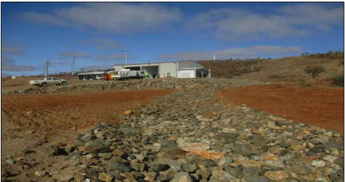
Photo: Operations and Maintenance Facility, with rehabilitation works commenced.
