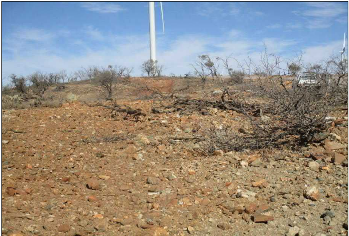
Photo: Underground HV electrical trench between overhead line and T52: Rehabilitation complete.
