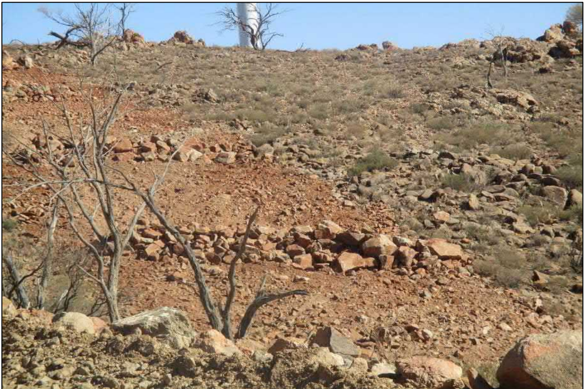
Photo: Underground HV electrical trench between T07 and T08: Rehabilitated with rock barriers or diversion banks installed to control and disperse any downhill water flow.
