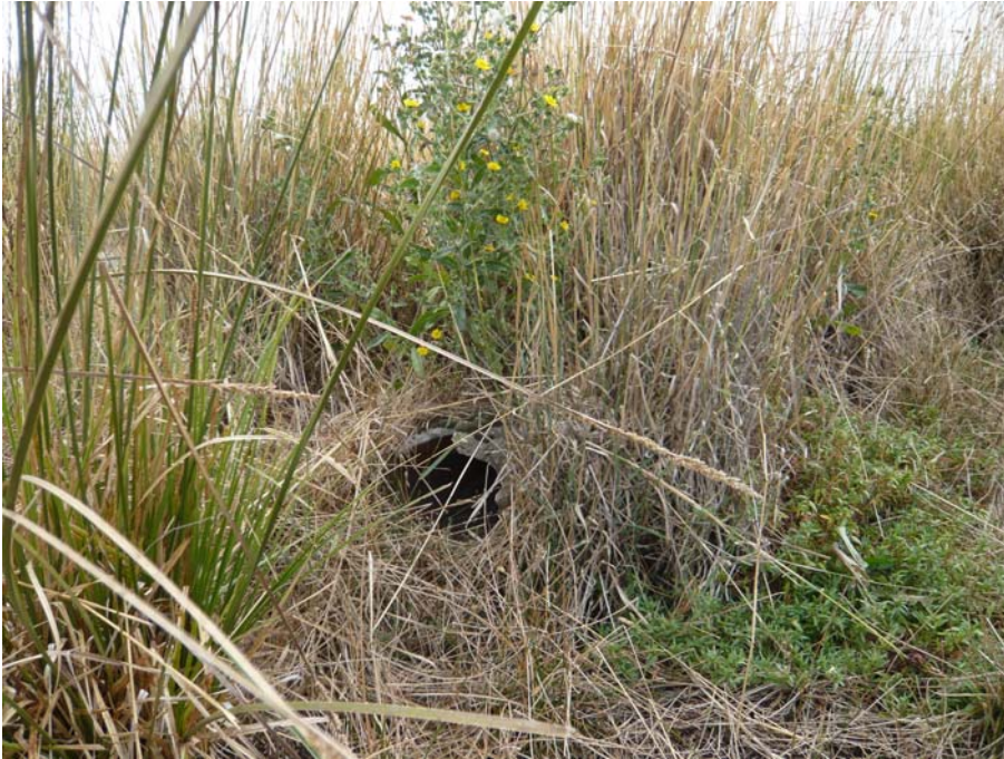
Plate A-3 Pipe culvert (note apparent flood debris), 28/2/2009
