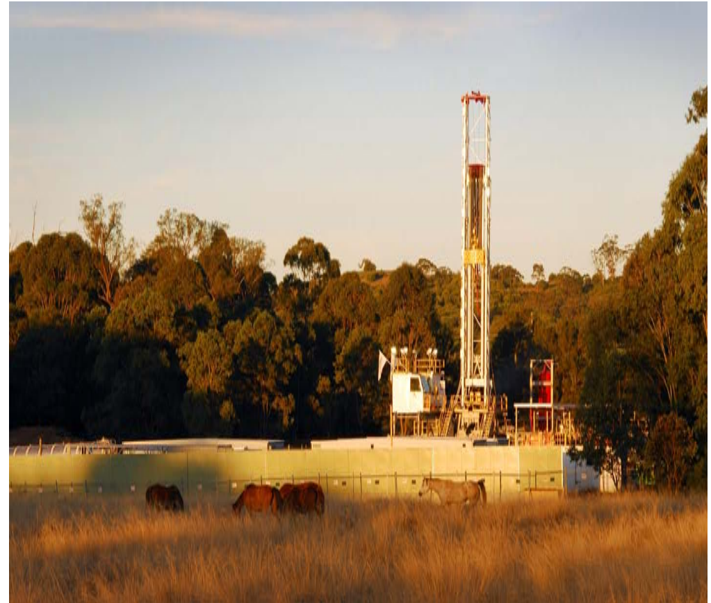
Ensign Rig 67 – ADR 200: automated and silenced to work in a semi urban area
