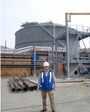
Gas storage facility
