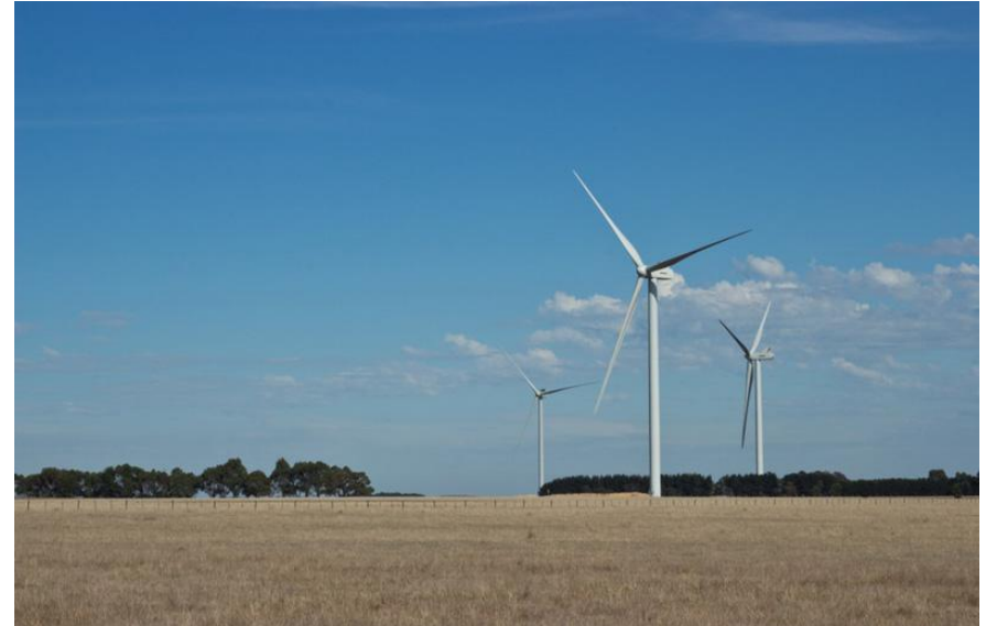
Macarthur Wind Farm under construction
