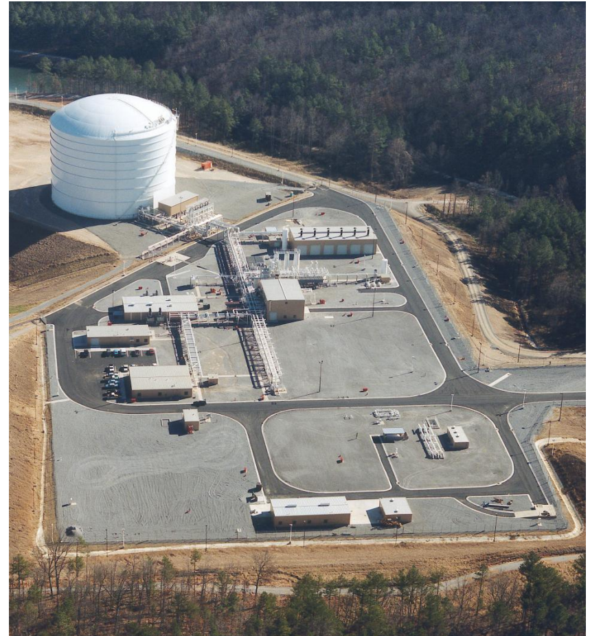
A similar facility in the USA (photo courtesy of CBI)
