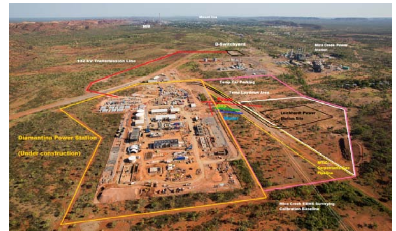
Aerial image of Diamantina Power Station site
